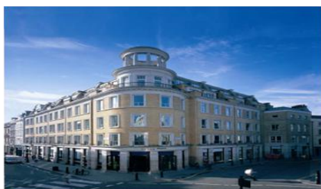
7. 21-25 Bedford Street & 20-22 King Street, London
