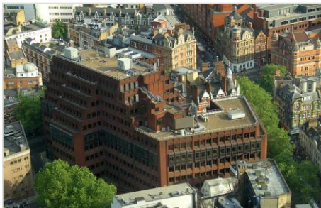
3. 125 Shaftesbury Avenue, London
